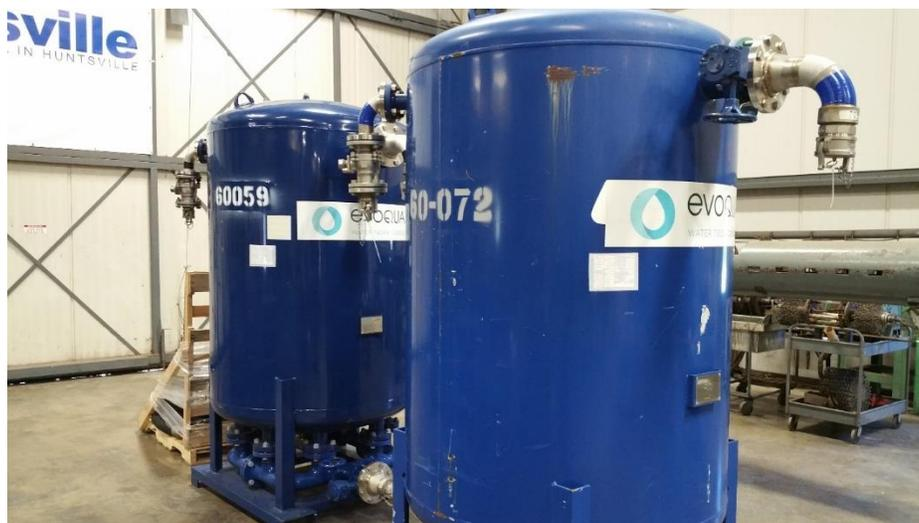
**FIGURE 5.** Deionization tanks for the water system.
